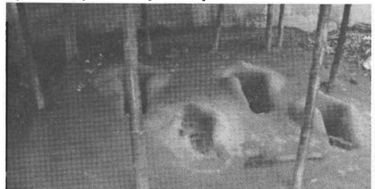
This Is A Scene Of The Cooking Area (Kitchen As We Know It). Where Most Of The Cooking Is Done. It Is To The Rear Of The Hostel In An Open Area With A Grass Roof Held Up By Bamboo Poles. There Are Four Holes In The Ground Which Are Lined With Cement. A Fire Is Built In The Hole And The Cooking Containers Are Placed On Top.
